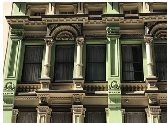
18 Detail view of moulded detailing to pilasters and columns Source: City of Sydney Council, August 2020
