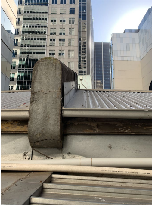
19 View of corrugated metal roof to 15-17 Hunter Street
