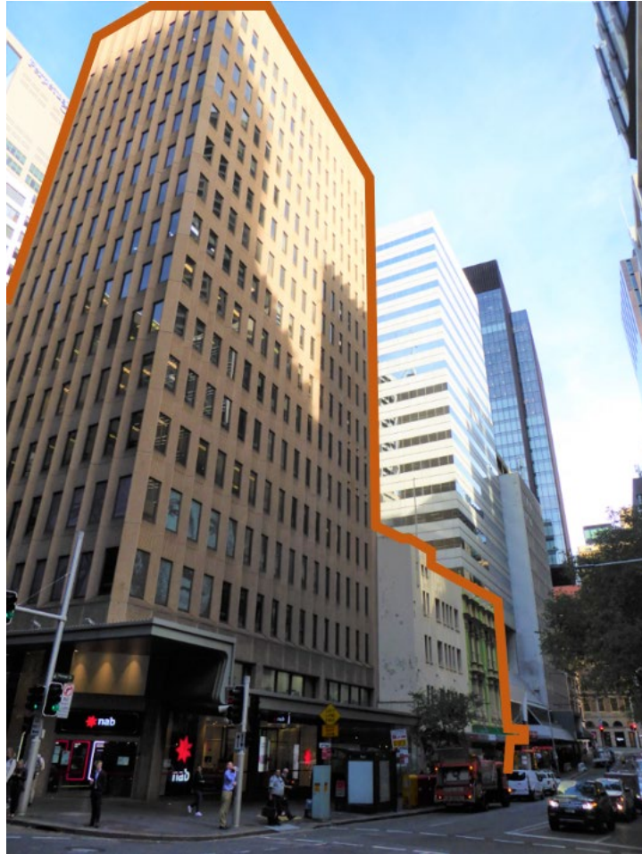
Figure 4. Subject site on the corner of Hunter and Pitt Streets, looking west along Hunter Street
