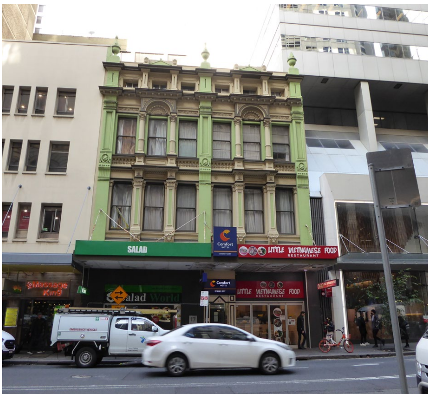
Figure 15. Pangas House at 15-17 Hunter Street
