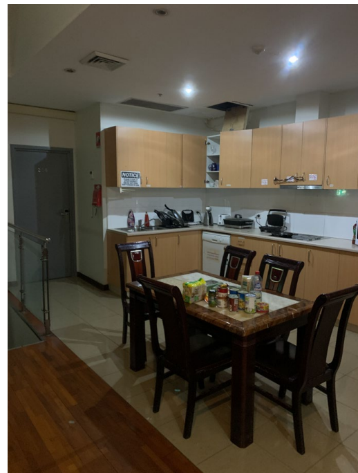
24 View of interior fitout showing low-height ceiling concealing services
