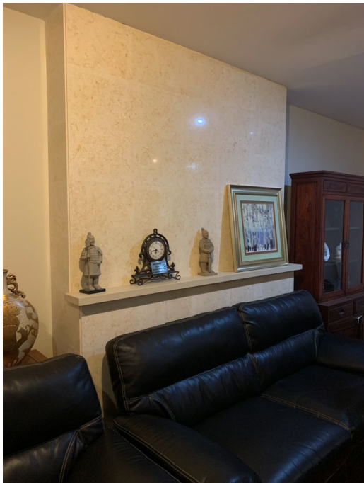
27 View of interior fitout and projected wall, within lining behind, possibly concealing early evidence of fireplace.
